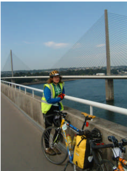
Crossing the Pont Albert Loupe into Brest.
